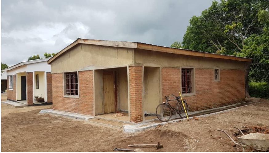
Photo 6. Construction of Nurse's House on site
